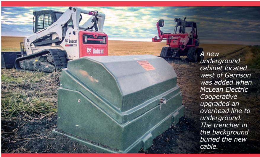
*A new underground cabinet located west of Garrison was added when McLean Electric Cooperative upgraded an overhead line to underground. The trencher in the background buried the new cable.*
